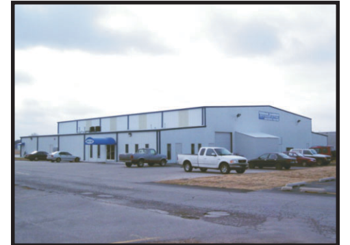
SWAS new 20,000 sq. ft. facility at RVS.
