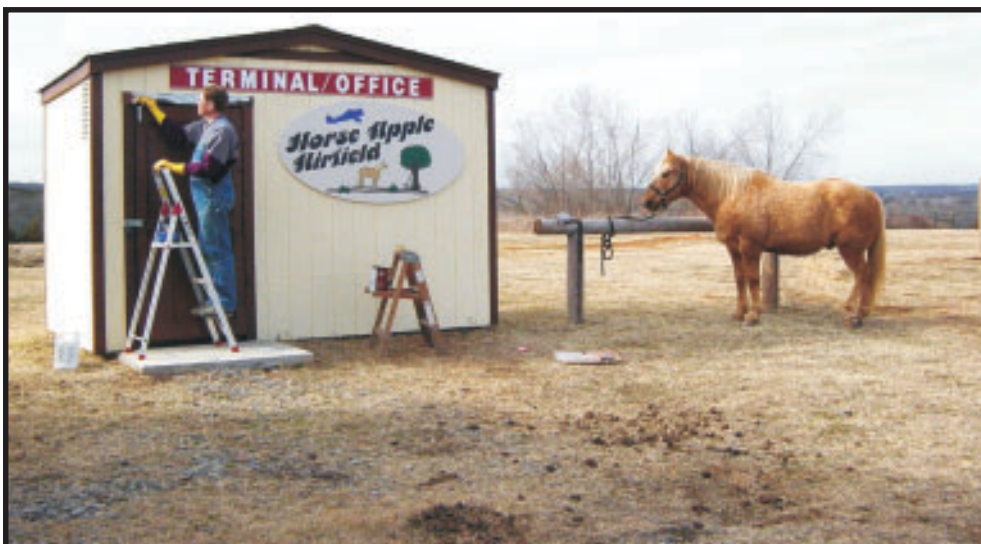
The newly remodeled HAA terminal building. The "courtesy car" awaits at the rail.
